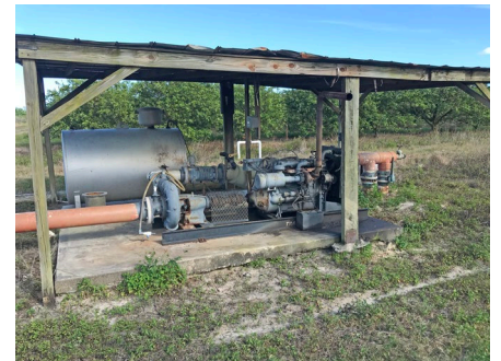
Diesel Irrigation Pumps
