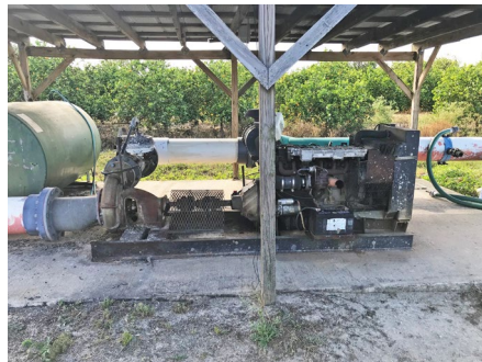
Diesel Irrigation Pumps
